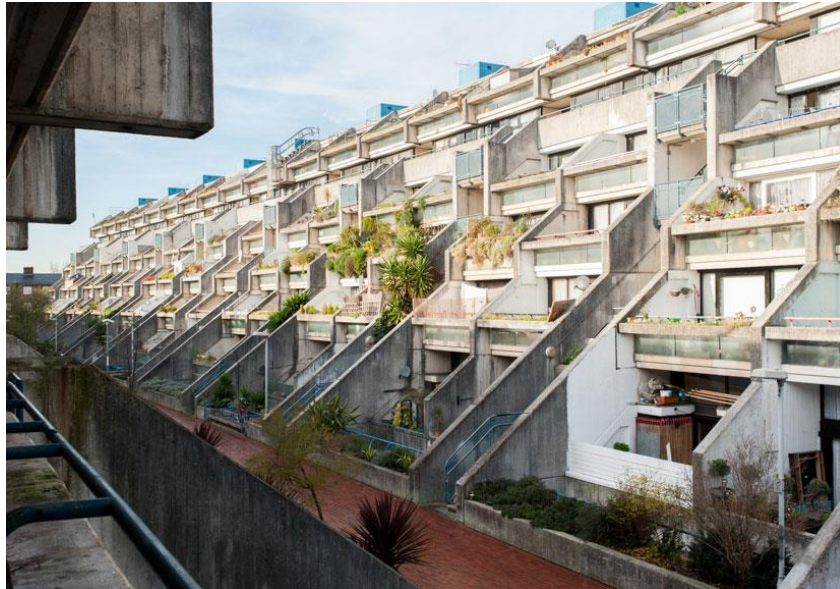
Figura 09: Alexandra Road / London Borough of Camden (1968) - Neave Brown
